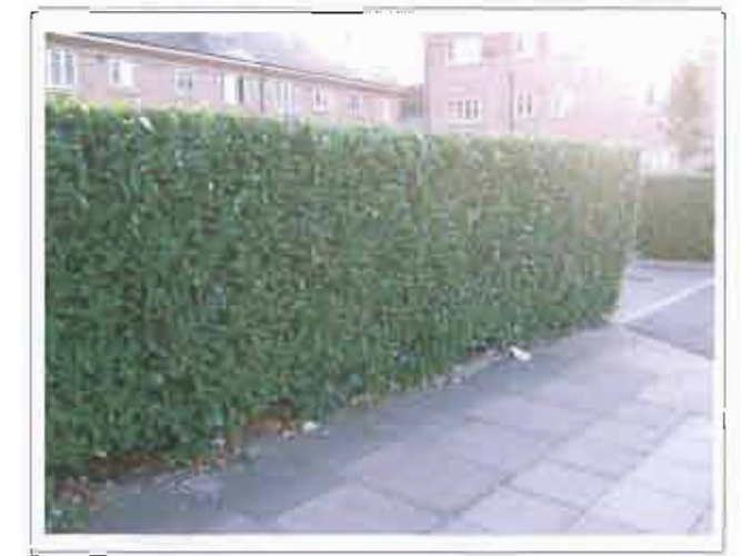
HEDGE GROWN THROUGH RAILING AS BOUNDARY TREATMENT
